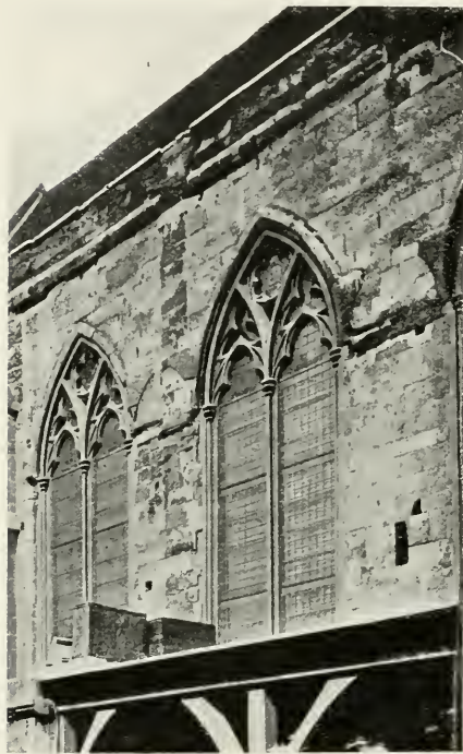
47. Side Windows, St Etheldreda, Ely Place.
